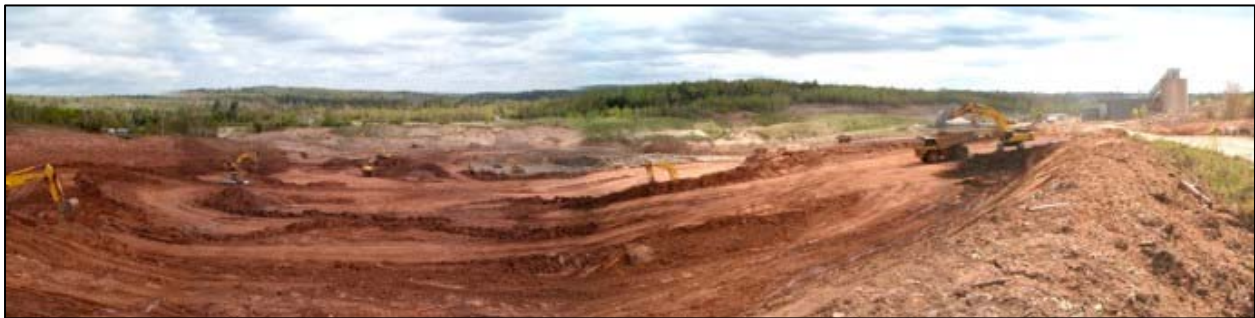
Scotia Mine, Gays River, June 1 st , 2007: Sand on top of the zinc-lead ore is being removed.
